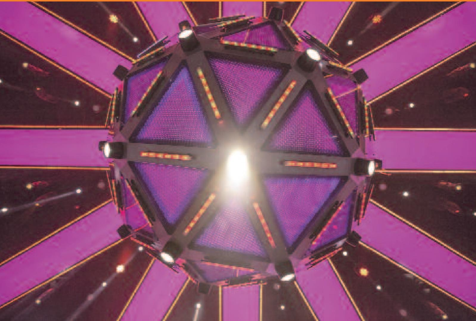
The Drai's disco ball incorporates 80 triangular segments that include 12" RGB LED Philips Color Kinetics iCove QLX LED strips as perimeter lighting around each triangle. At each triangular intersection is an Eurolite pinspot and filling in the interior space of each triangle is a small 10mm SMD LED video tile.
