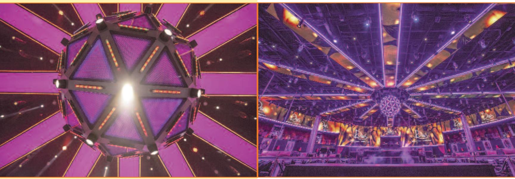
The Drai's disco ball incorporates 80 triangular segments that include 12" RGB LED Philips Color Kinetics iCove QLX LED strips as perimeter lighting around each triangle. At each triangular intersection is an Eurolite pinspot and filling in the interior space of each tri-angle is a small 10mm SMD LED video tile.
